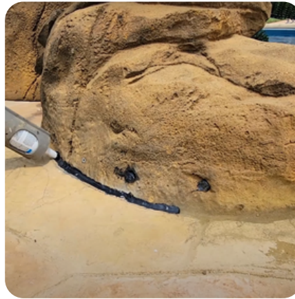
Now apply silicone or M-1 around the edges and screw heads.
