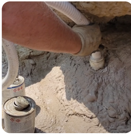
Glue the flex pipe into the fitting.
