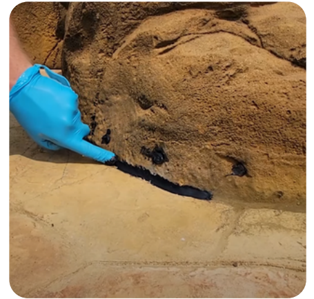
Use a glove to spread the silicone evenly as shown.
