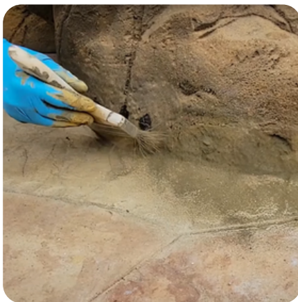
Using a paintbrush, dip it into the powdered coloring and apply it directly to the wet silicone, effectively camouflaging the spots.
