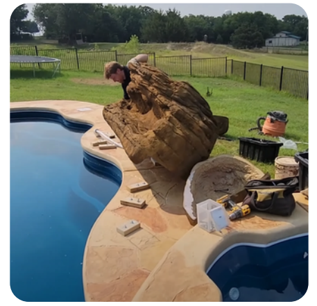
Insert all the flex pipe into the waterfall, then carefully flip the waterfall and rocks over. Position them correctly over the mounted blocks and test water flow.
