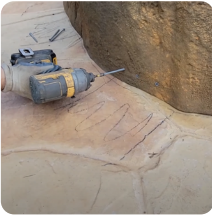
After testing the water flow and ensuring it operates correctly, switch off the waterfall. Next, use the marked lines as a reference to secure screws through the exterior of the rocks into the blocks beneath.
