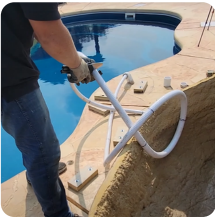
Cut off the excess flex pipe.
